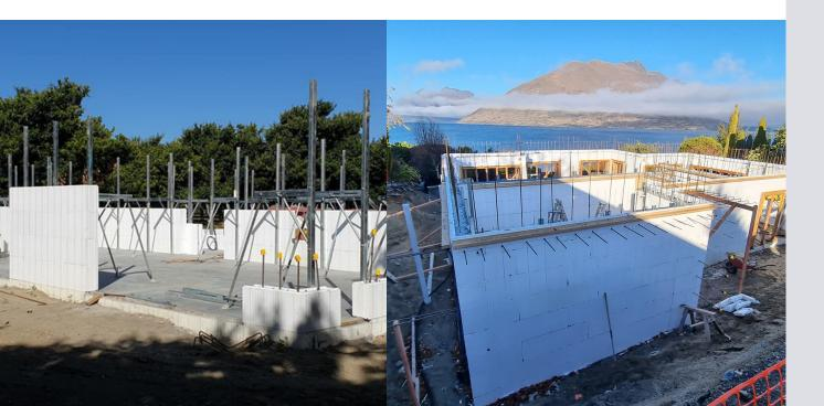
Insulated Concrete Formwork, or ICF, are hollow and lightweight insulated forms that are erected at the construction site. The forms are easy to assemble due to their lightweight material and are stacked on top of each other onsite. The forms are filled with 150mm of poured-in-place, waterproofed, reinforced concrete. Unlike traditional concrete forms, which are removed after the concrete cures, ICFs are left in place.
